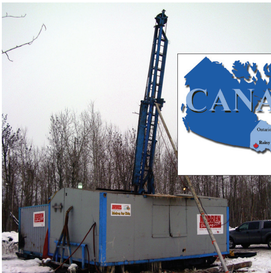
Drilling continues on Bayfield Venture's Burns Block.
